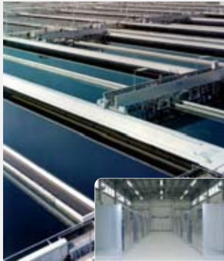
• Sewage purification ROBOX evolution blower unit
